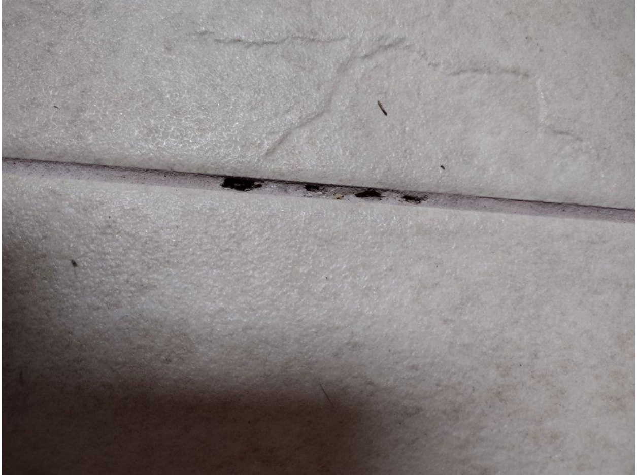
Grout holes, Photo 2.
